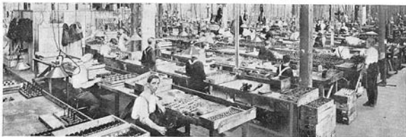
FIG. 61.—ASSEMBLING HOOKSWITCHES AND TRANSMITTER ARMS
