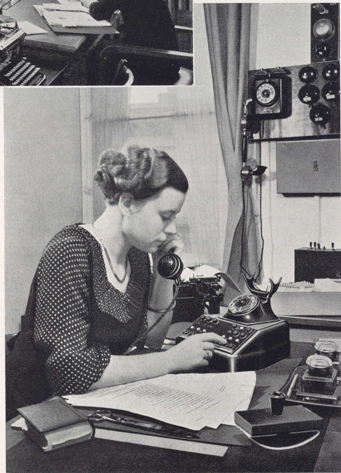
Operator's Position of a NEHA Private Exchange equipped with 3 exchange lines and capable of connecting up a maximum of 25 extensions
